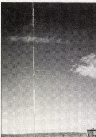
Fig. 4: This 200ft tower holds a 'six over six' for 14MHz and is John's largest tower.
