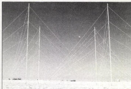
Fig. 2: John Brosnahan W0UN's 'four square' array for 1.8MHz consisting of four towers, 160ft high, fed as verticals.
